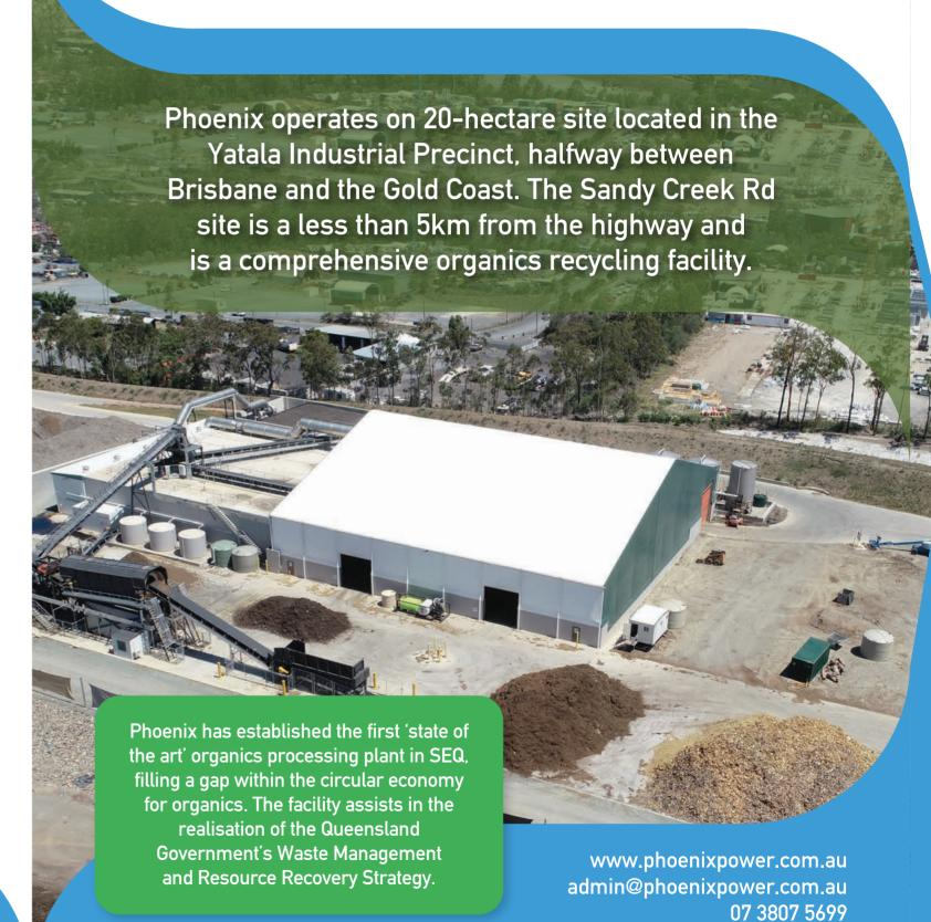
Utilising advanced manufacturing technology and best practice recycling methodologies, the site runs four fully enclosed aerated-floor composting vessels. The receival hall is under negative pressure to ensure there are no emissions from wastes with potential for nuisance odour.
